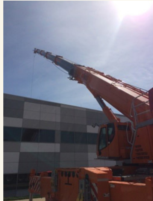
PSC lifts HVAC units on to rooftop
